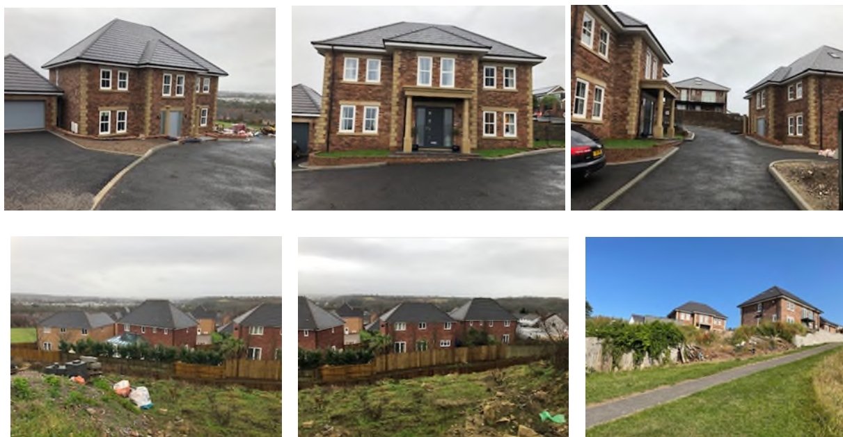
Fig. 5 – Photographs of the application site
